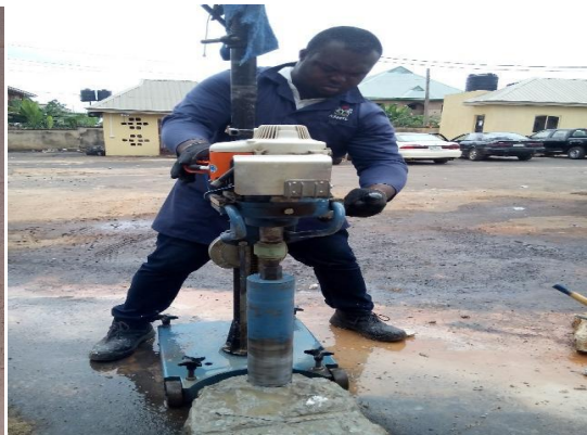
Plate 3. Coring of the concrete mass sample
